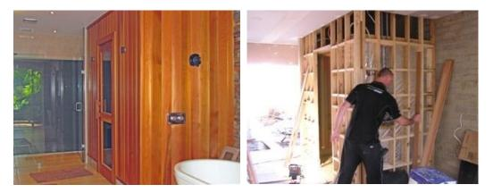
The sauna is a wooden stud and frame construction, clad on the inside and outside with Western Red Cedar panelling, and with foil and fibre insulation. The photographs shows the sauna under construction, and the Feonic audio drives were mounted on the outside of the sauna walls after they were completed.
